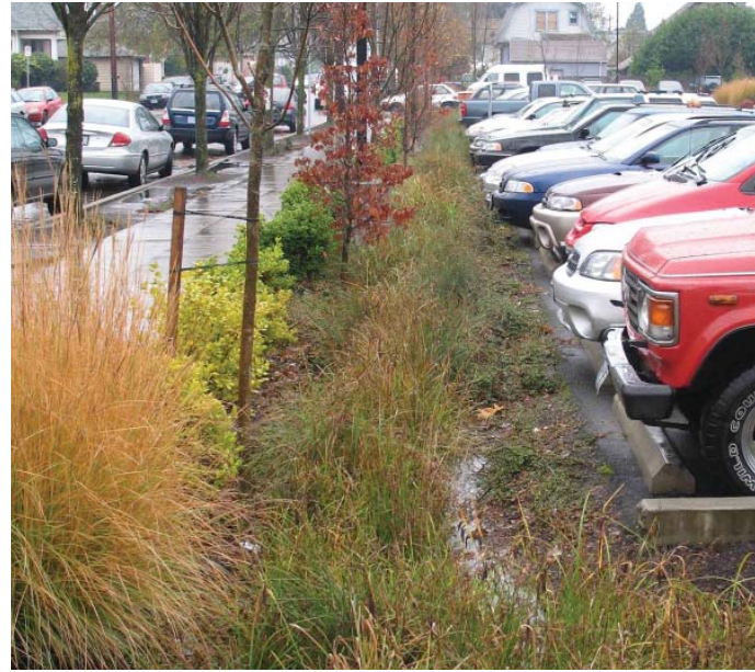
On-site stormwater management at surface parking lots and along streets will reduce runoff while beautifying the environment.
